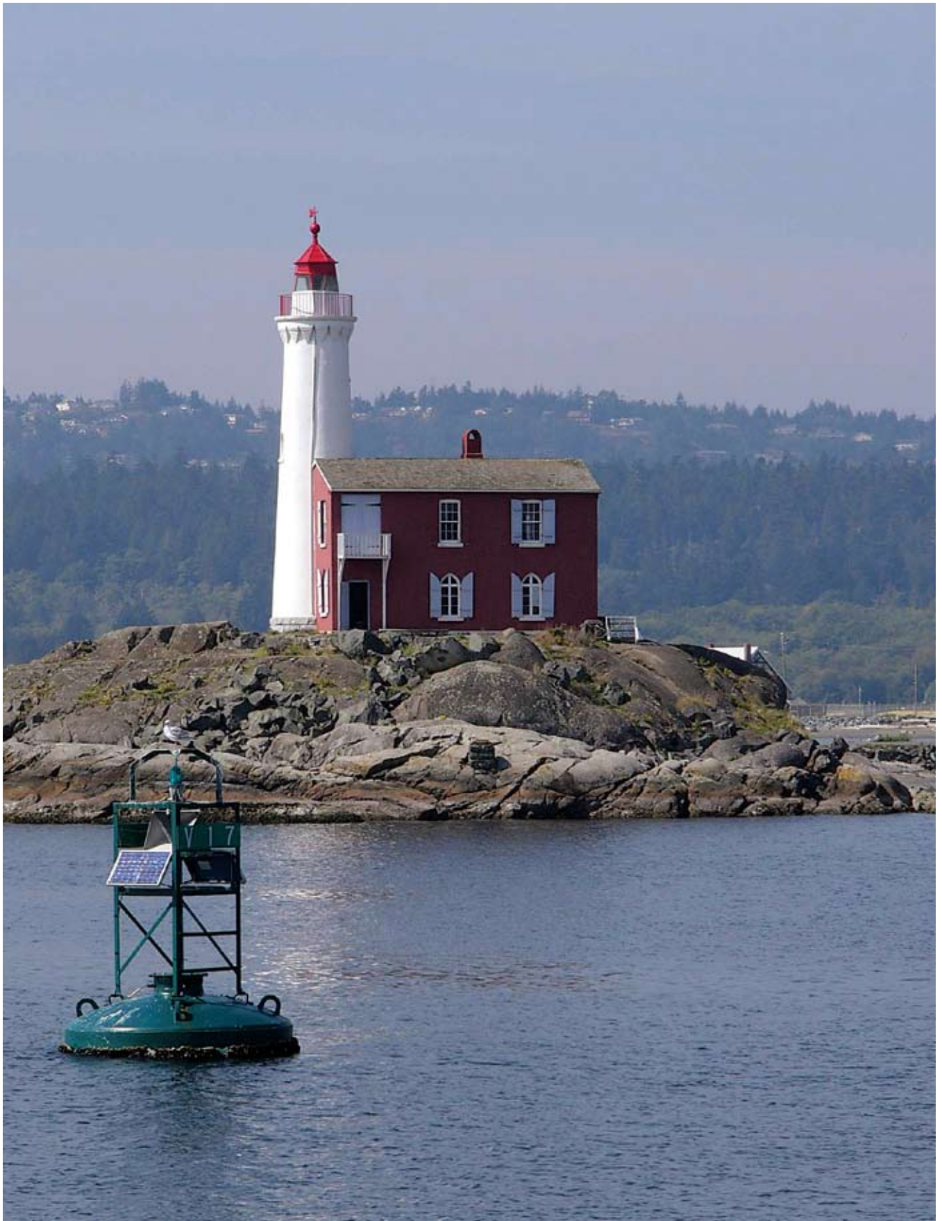
The Fisgard Lighthouse National Historic Site at the mouth to Esquimalt Harbour commemorates the first lighthouse on Canada's West Coast.
